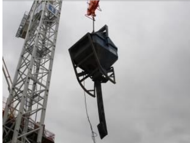
Double jubilee clips & fall arrest chain if tremmie tube fitted
