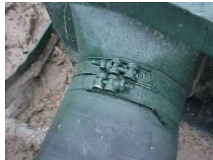
Double jubilee clips & fall arrest chain if tremmie tube fitted
